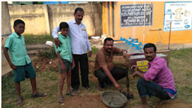
A handwash station being installed at a government primary school.
