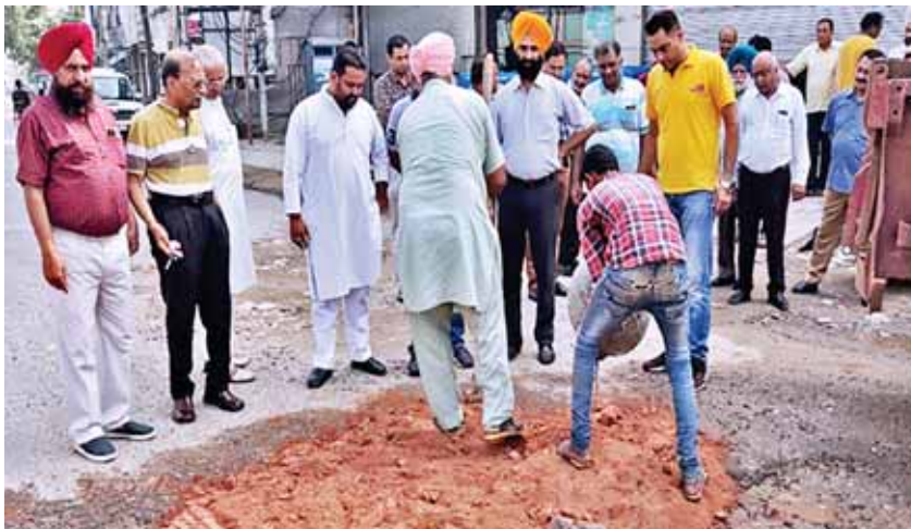
Rotarians do patch-up work on damaged roads.
