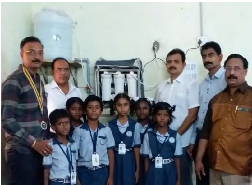
An RO plant installed at a government school.
