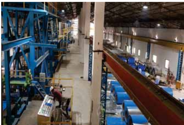
Colour coating Plant at Umbergaon, Gujarat
