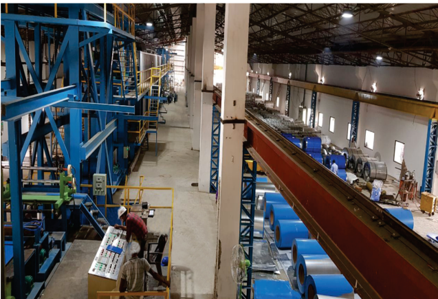
Colour coating Plant at Umbergaon, Gujarat
