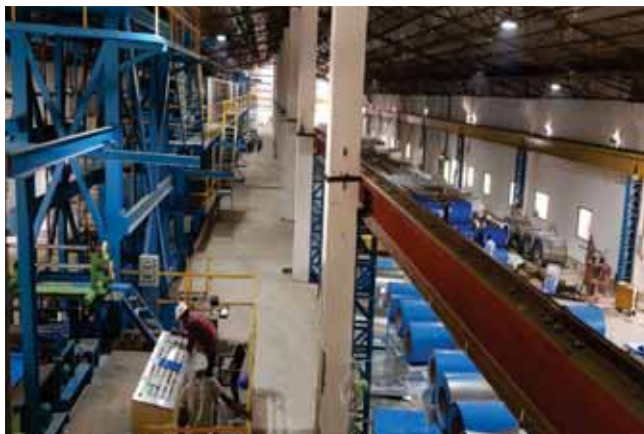
Colour coating Plant at Umbergaon, Gujarat
