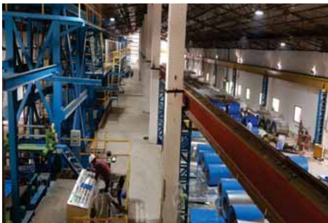
Colour coating Plant at Umbergaon, Gujarat
