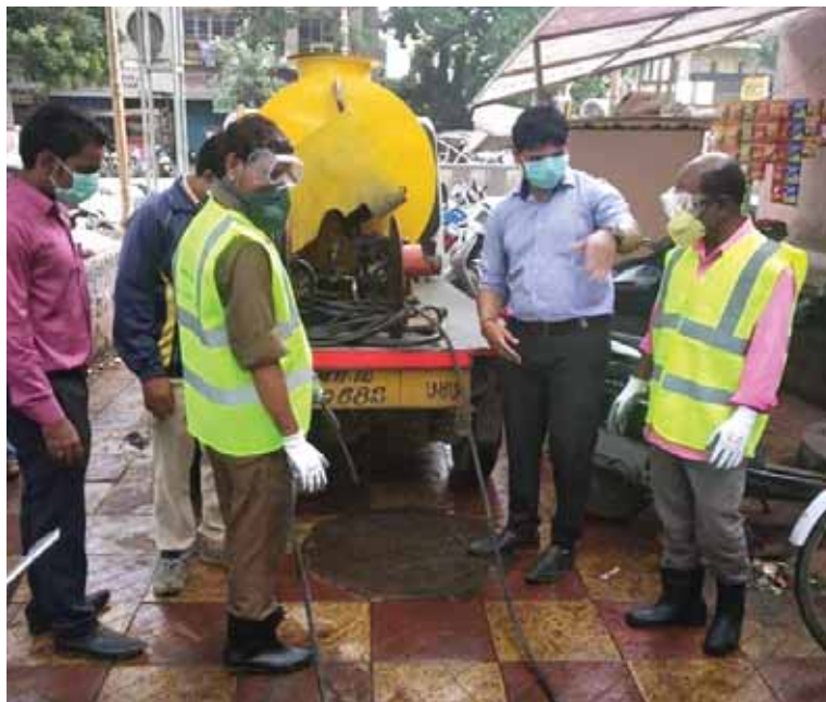
Sanitation work in progress.
