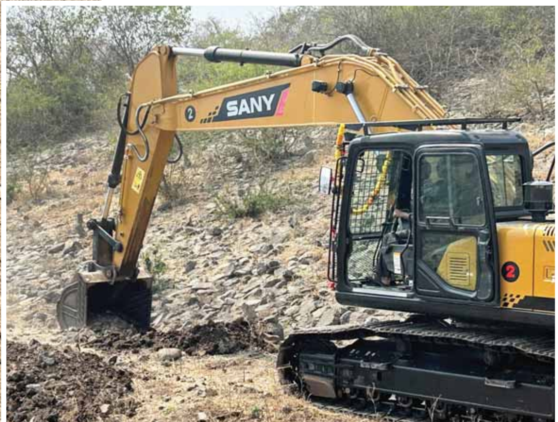
A trench being dug at the dam site.
