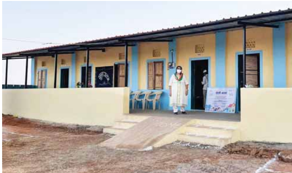
The renovated classrooms.
