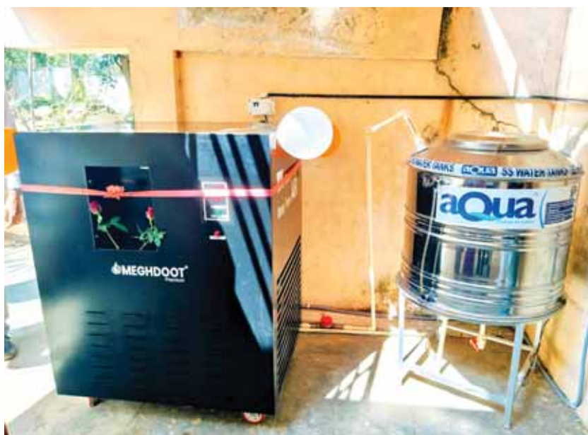
The newly installed AWG kiosk.
