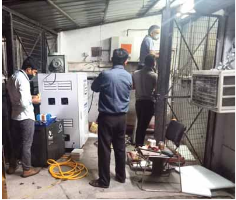
An oxygen generating plant being installed at a hospital in Delhi.
