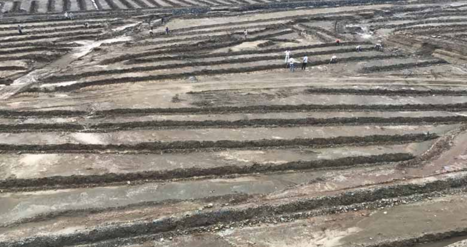
Trenches made on the ground to hold water.
