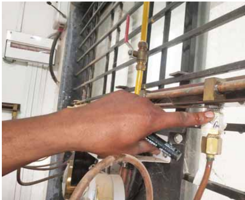
An ultrasonic machine being used to detect and plug leakage in an oxygen pipeline.
